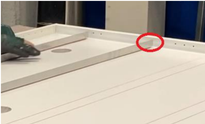
Figure 7 Pointing the gap between reinforcement part and the edge of ceiling
